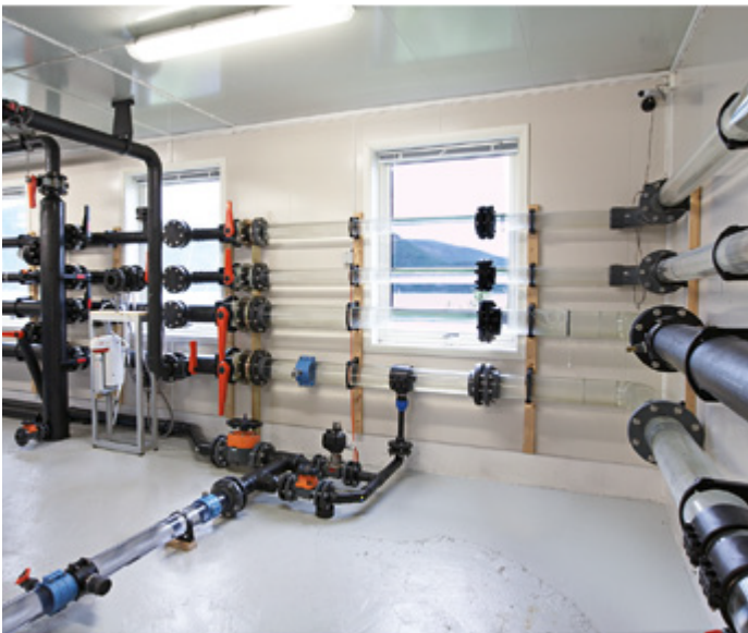
Transparent pipework to visualise optimum gas dissolution
